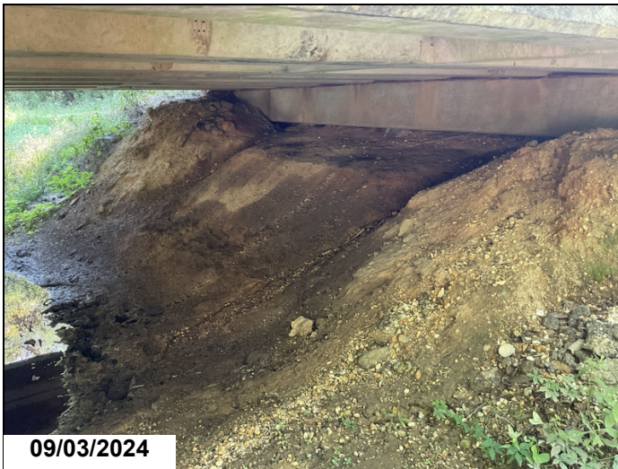
Abutments 2 slope has a large scour hole from pile 2 - 4.
